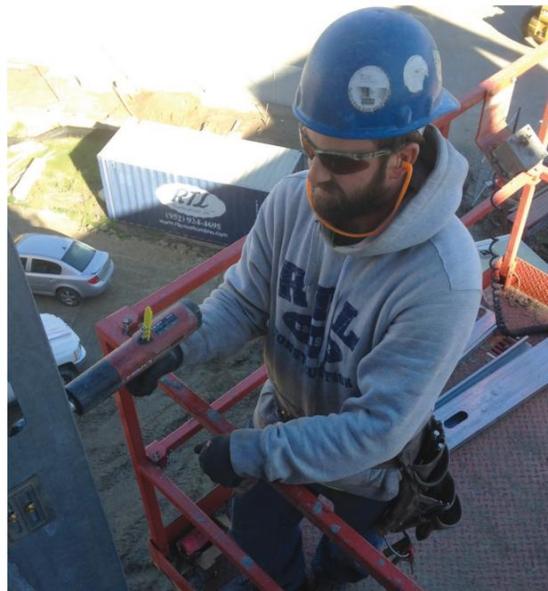
**There are many uses for powder actuated fasteners in the field. RTL Construction will provide further training sometime after the first of the year to further ensure safe practices when using these high powered tools.**
